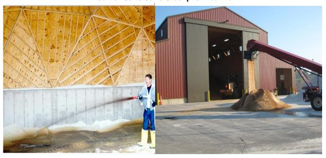
Apply at 4-5 gals/ton (15-19 liters / metric ton) Reduce application rate 30% Freeze point -40°F (-40°C) Reduce Operating Cost Reduce bounce and scatter loss PDSgeo55-042414 Apply at 55% solids no need to dilute with Brines Prevents freezing, crusting – salt free flowing Truck and Employee can cover 30% more area Reduced corrosion
